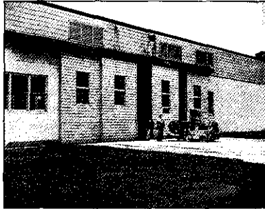
Building 105, Area C, May 1952.
