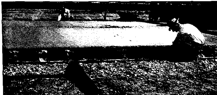
Construction of Wright Field runways in August 1944.
