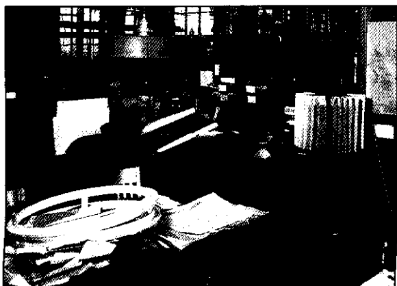
Machine Shop office, McCook Field.
