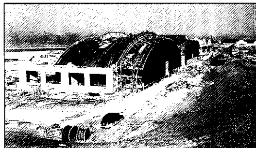
Hangar 4 under construction.
