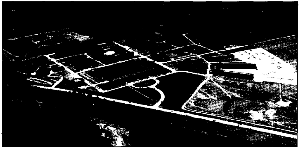
Aerial view of Wright Field, September 1939.
