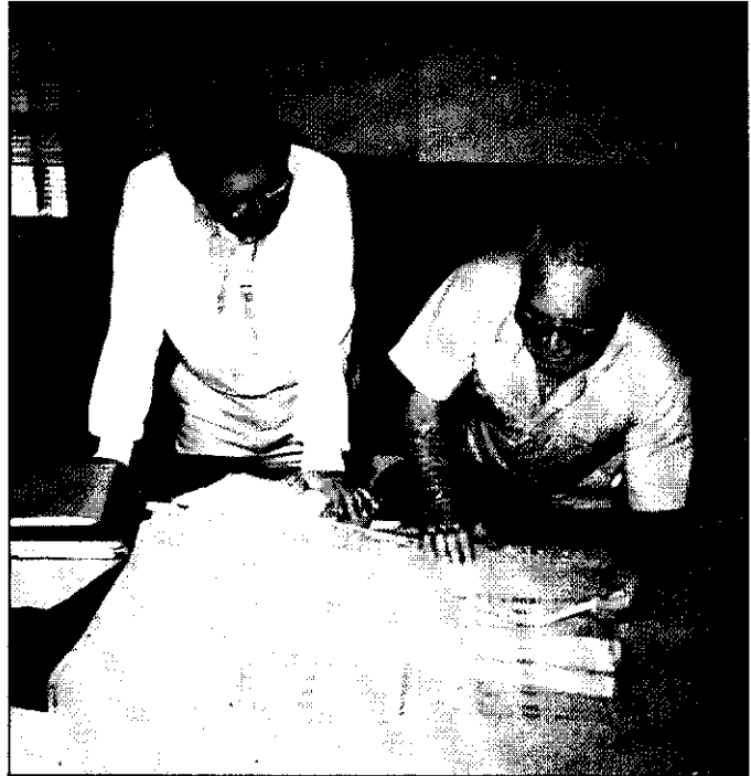
Reviewing instrumentation installation drawings, ca. 1985.
